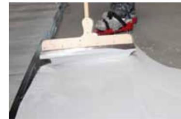
12. Apply the LF-VL with a slotted squeegee or trowel in two layers. Consumption per mm layer thickness is 1.3 kg per m<sup>2</sup>.
