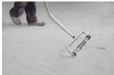
4. When shot blasting is performed with steel abrasive, the surface is cleaned with a magnetic broom. The collected shot can be re-used.
