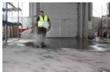
8. Broadcast dried silica sand into the wet primer (only when primed with KÖSTER LF-BM) to increase the bond strength of the subsequent layer.
