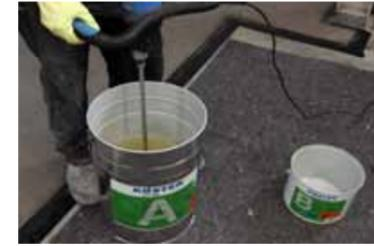
10. The components are mixed for a minimum of 3 minutes with a mechanical stirring device until a homogeneous consistency is reached. Follow the mixing procedures given in the Technical Guideline.
