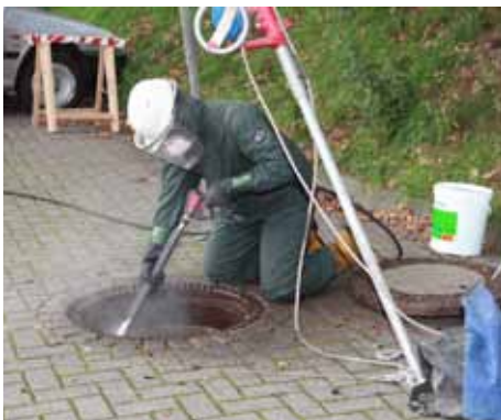
Substrate preparation (In this case high pressure water jetting)
