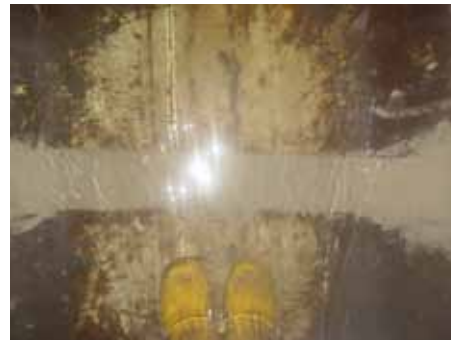
Very stable - even under flowing water
