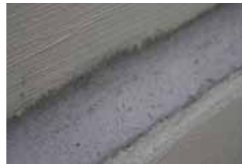
2. Fillet installed with KÖSTER Repair Mortar
